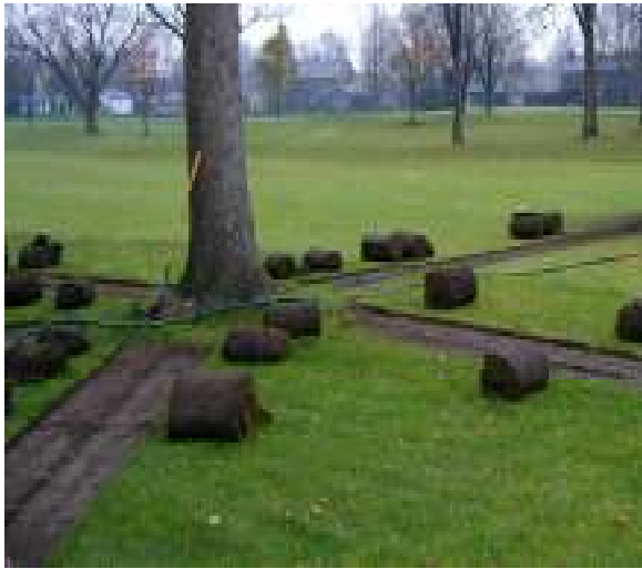
Sod cut and rolled for reuse.
